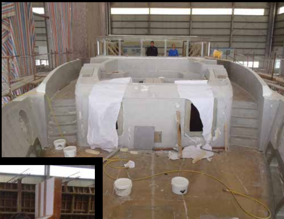
Captain Bryan Carter, left, gets a sense of things from the pilothouse during "decking down" of the upper deck. Off the captain's right shoulder can be seen the author's project manager office, built just astern of the vessel.
